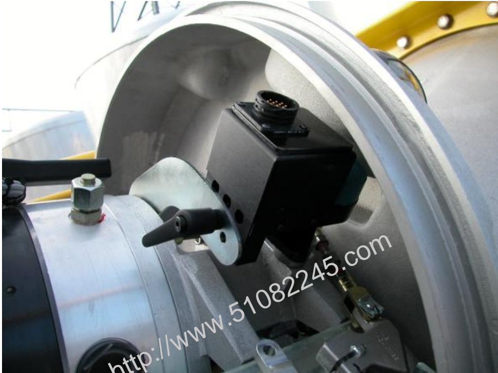
Rotary Transducer on ABB HMB Mechanism
