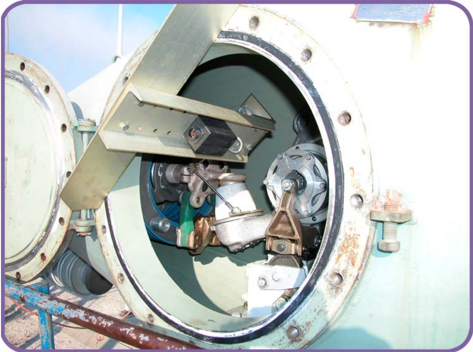
Figure 29. Westinghouse SFA Transducer Installation
