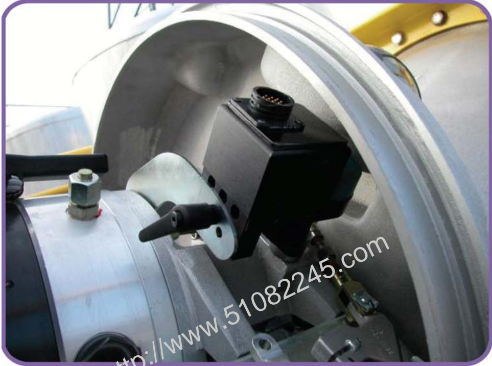
Figure 28. Rotary Transducer on ABB HMB Mech
